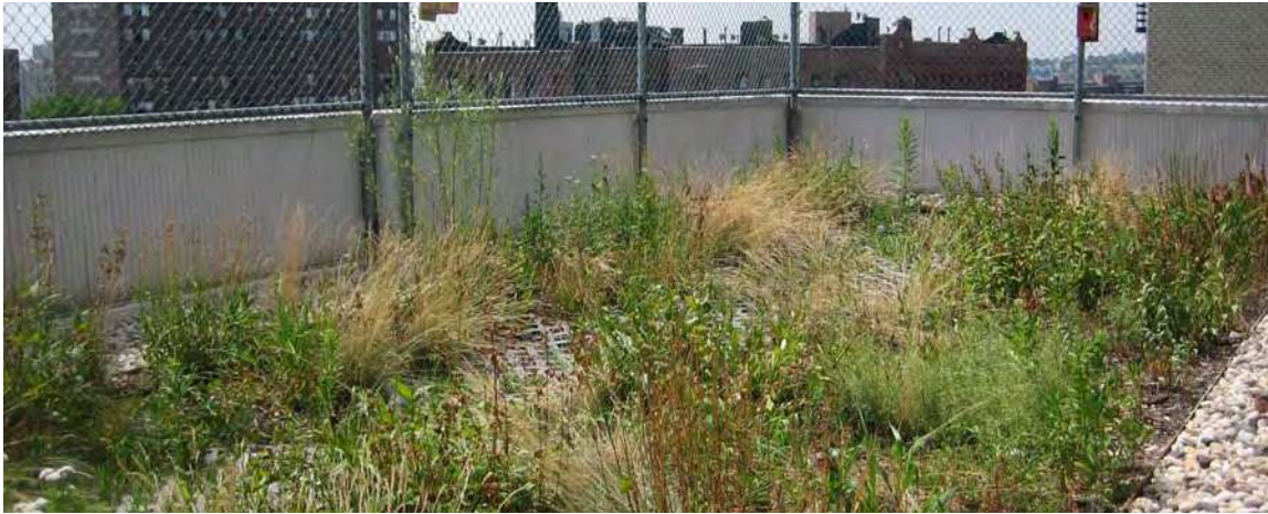
Figure 4-18: Fence installed on St. Simon Stock School in the Bronx to allow student access to the green roof.
