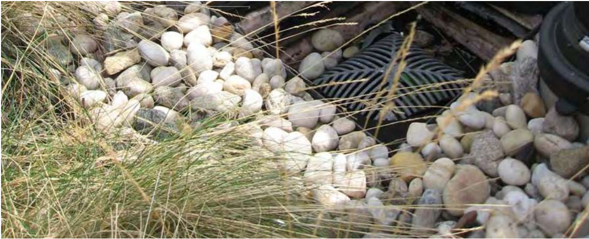
Figure 4-21: Green roof drain inspection cham- ber on St. Simon Stock School in the Bronx.
