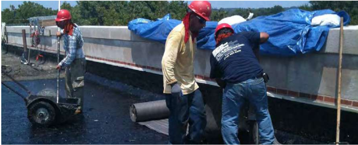
Figure 4-15: Application of tar and waterproofing membrane during installation of a green roof at PS118 in Queens.
