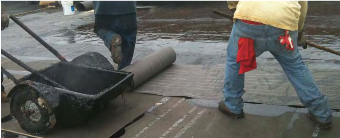
Figure 4-8: Installation of fiberboard and first ply of waterproofing membrane during construction of a blue roof at PS118 in Queens.
