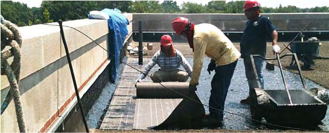
Figure 4-9: Installation of waterproofing membrane during construction of a green roof at PS118 in Queens.
