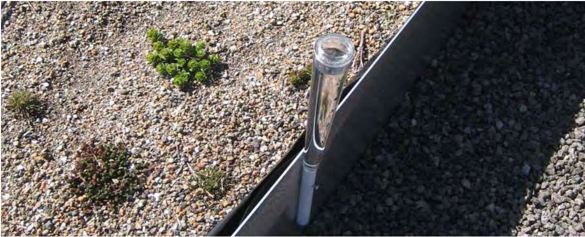
Figure 4-20: Rain gauge at PS118 in Queens.
