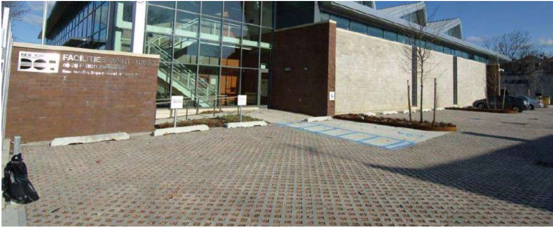
Figure 3-10: Permeable pavers installed outside a DOT maintenance facility in Queens.
