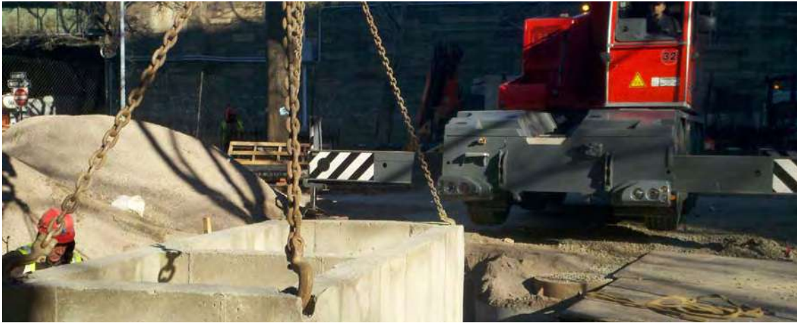
Figure 3-15: Pretreatment structures are typically installed after the geotextile and bedding stone is placed.
