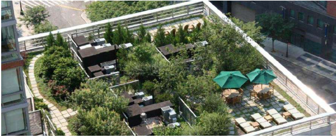
Figure 4-17: The green roof on The Verdesian, a residential building in lower Manhattan, provides dedicated space for access, passive recreation and the building's mechanical equipment.
