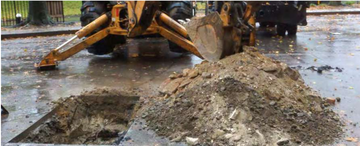
Figure 3-12: Test pits may be necessary to determine subsurface conditions, including potential soil contamination.
