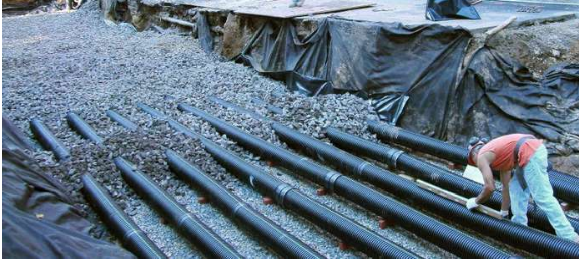
Figure 3-2: Construction of a perforated pipe system at NYCHA's Bronx River Houses in the Bronx.
