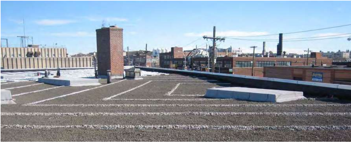
Figure 4-12: Intermediate check dams were installed on DEP’s Storage Facility in Brooklyn to control flow on sloped portions of the roof.
