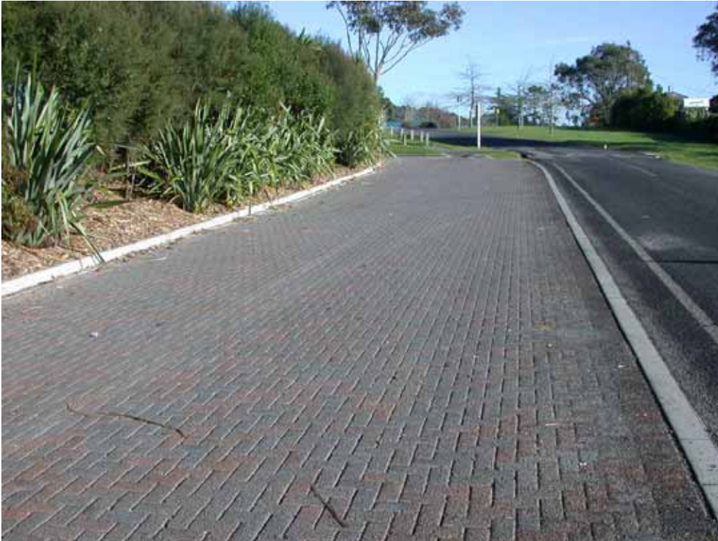
Figure 5.6 Permeable paving 'Formpave' at Parrs Park, Waitakere City
